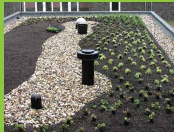
15. Impression of the green roof directly after construction.
