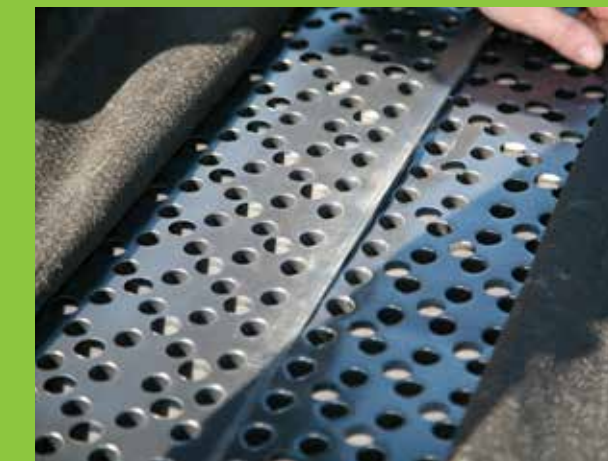
5. Place the ND Drainage System right next to the previous one.
