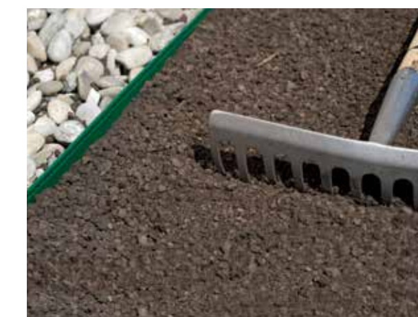
11. Divide the ND Substrate equally (5-8 cm).
