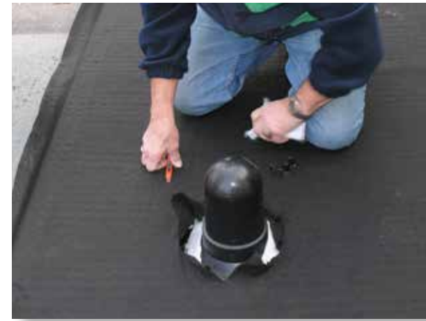
7. Cut out the roof outlets.
