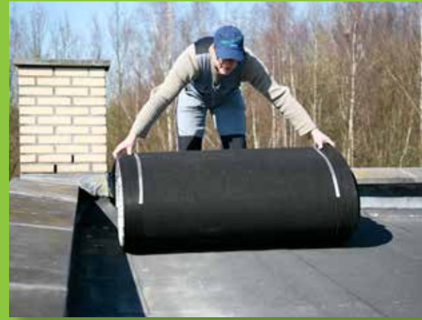
3. Position and unroll ND Drainage System.
