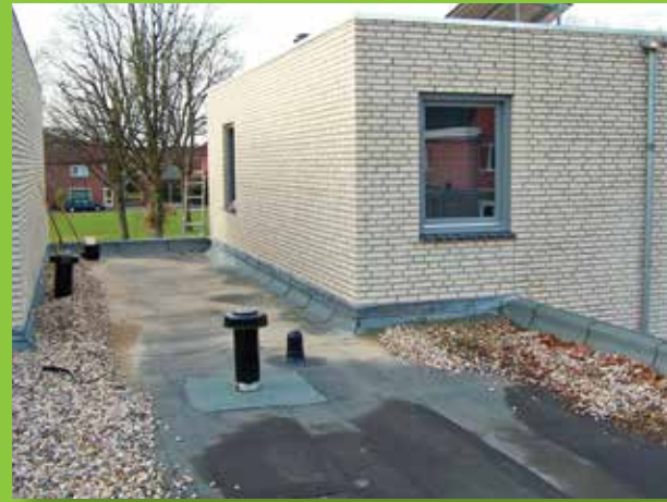
1. The Initial situation, a flat roof with bitumen roofing*.
