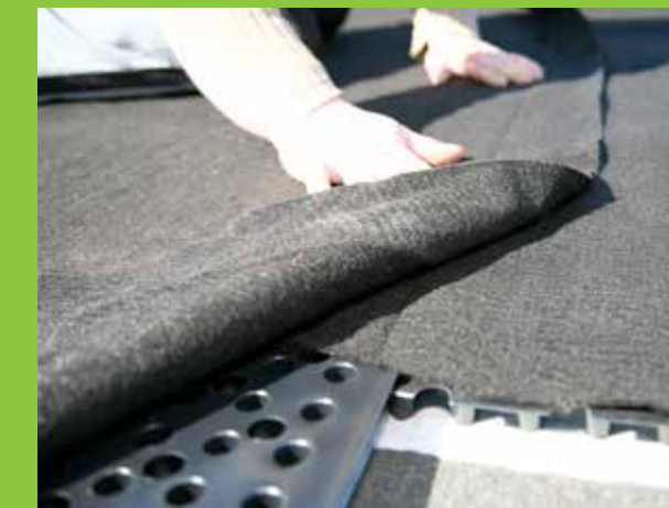
6. The filter geotextile has to overlap.
