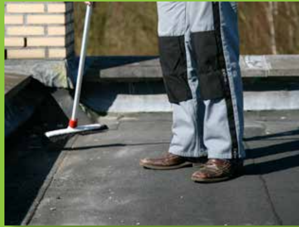
2. Clean roof with broom.
