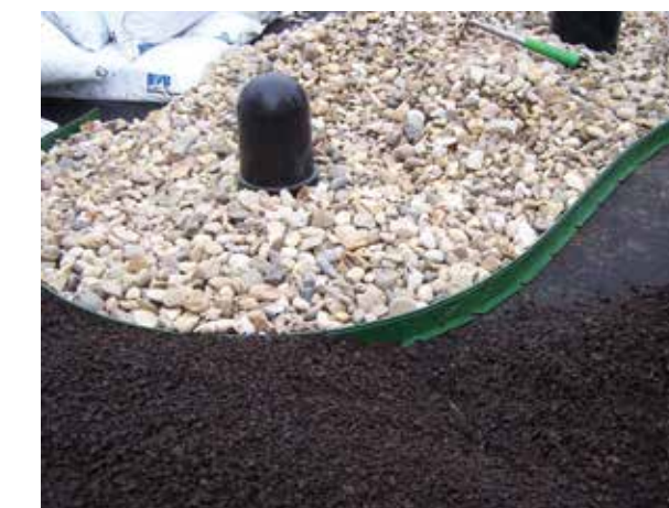
12. Create vegetation-free zones around roof outlets.
