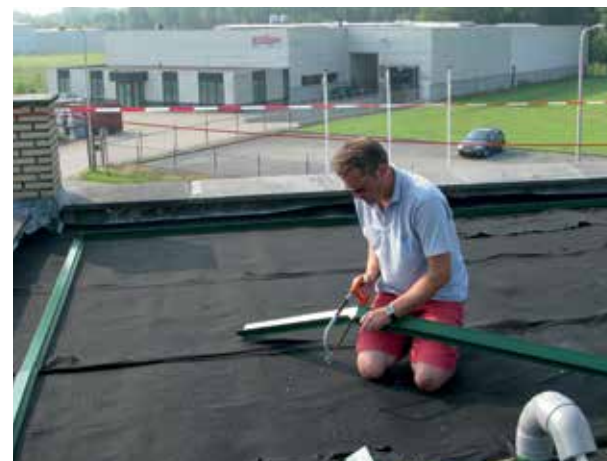
8. Install ND Edge Retaining Profiles.
